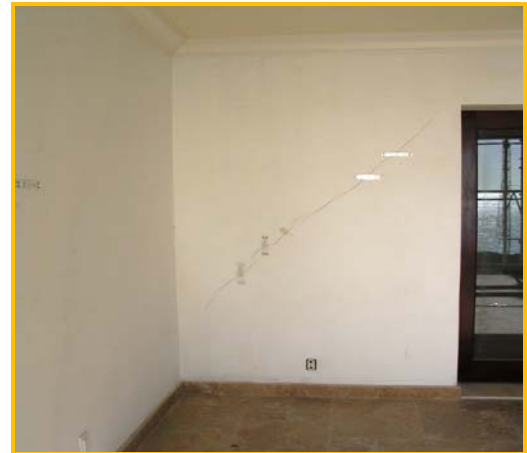
Figure 6: Interior Cracking
