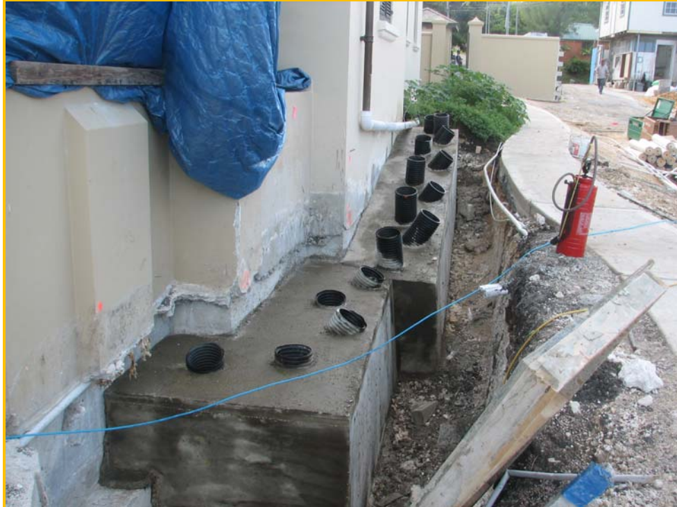
Figure 9: New Grade Beam around Foundation
