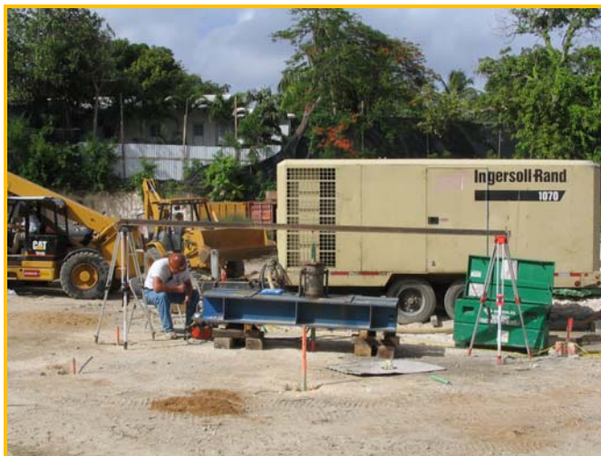
Figure 10: Micropile Tension Testing
