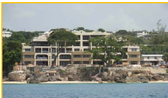
Figure 1: Sandy Cove Condominium
